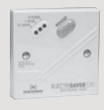
The towel radiators have temperature dials on them - these control how hot the radiators are to maintain a set temperature in the bathrooms - leave the dials set at number 3 for normal use. If you want to run them for a while when the heating isn't on, press the 'boost' switch on the landing.
