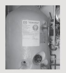
In summer the whole tank is heated up by the sun when it shines on the solar panels on the roof. In winter the sun heats the bottom half of the tank and the boiler heats up the top so you always have hot water even when three is no sun.
